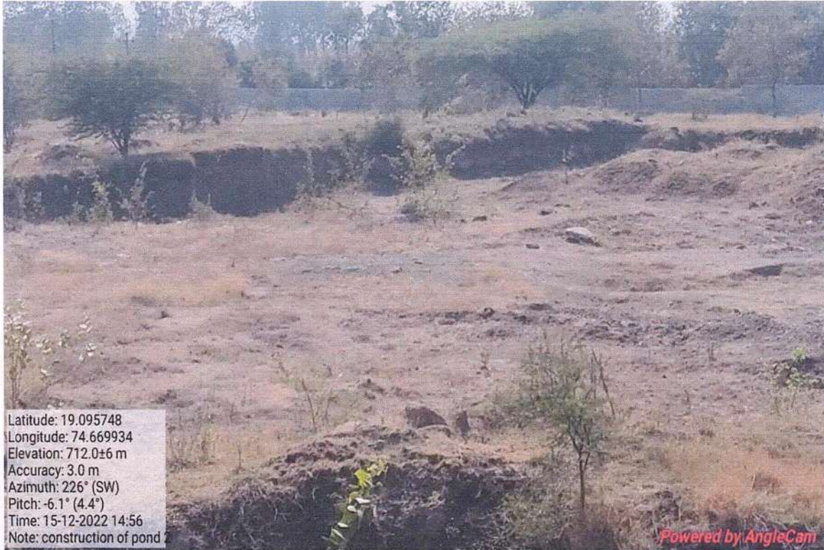
Image: Construction of pond
