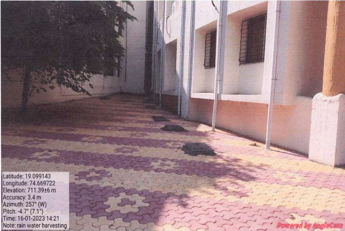
Image: Inspection Chamber
