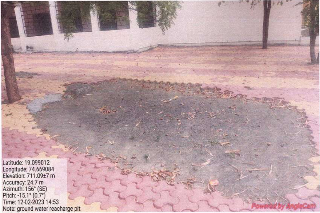
Image: Ground water recharge pit
